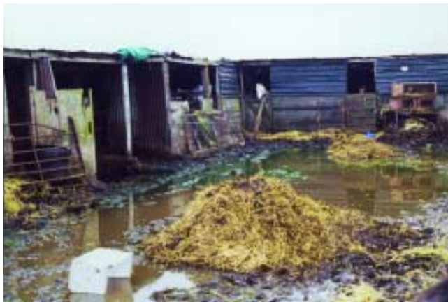
Fig 1: Full details and an accurate description of the premises must be carefully recorded.
